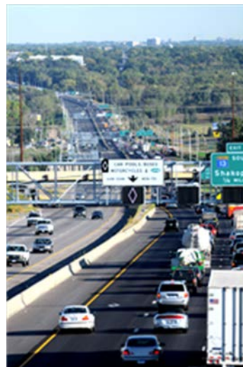
Figure MN-1. ATM signals on I-35W.
